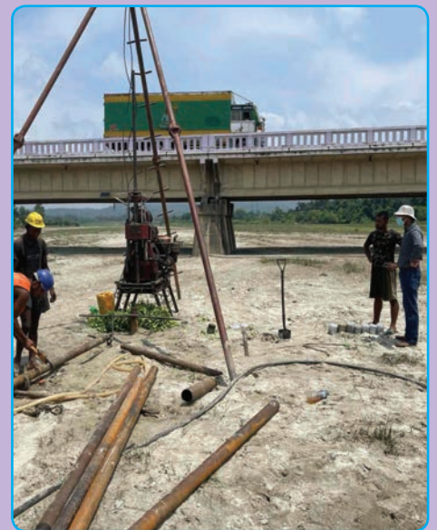
Field work Monitoring by Senior Geotechnical Engineer via Random Site Visit
