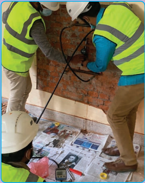
Flat Jack Test for Ritu Niwash at Manbhawan
