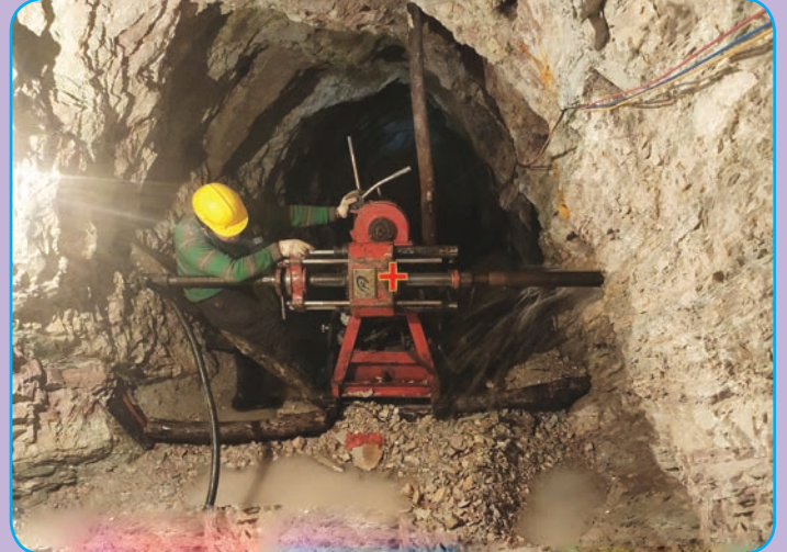
Horizontal Drilling inside Tunnel
