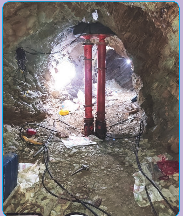
Plate Jacking Test inside Tunnel
