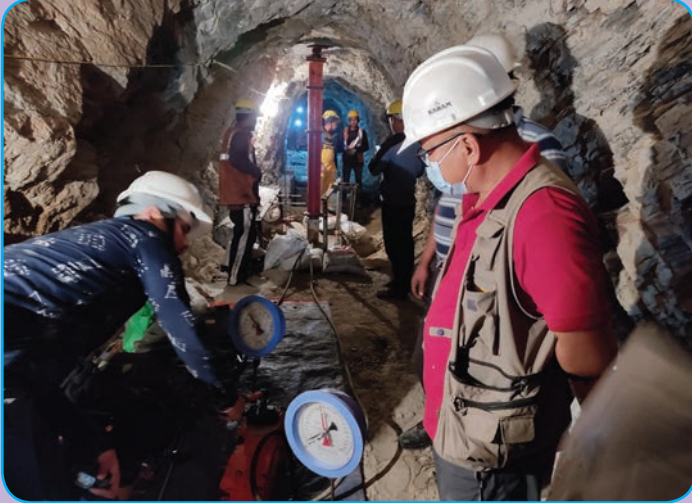
In-situ Direct Shear Test inside Tunnel
