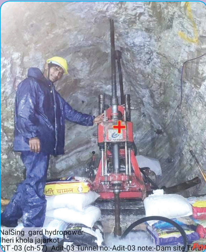
Vertically upward Drilling Inside Tunnel
