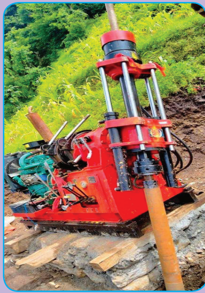
320m Rotary Drilling at KTFT Project with 1000m capacity Drilling Machine
