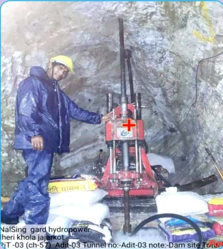
Vertically upward Drilling Inside Tunnel
