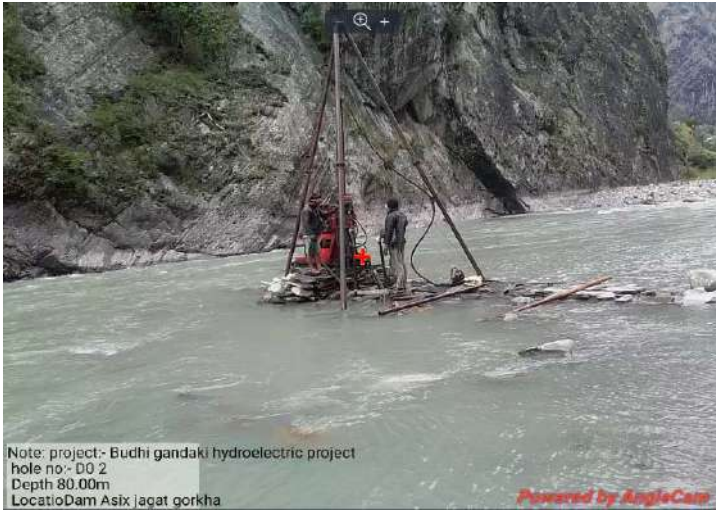
Fig: Budhi Gandaki Hydropower Soil Investigation Project
