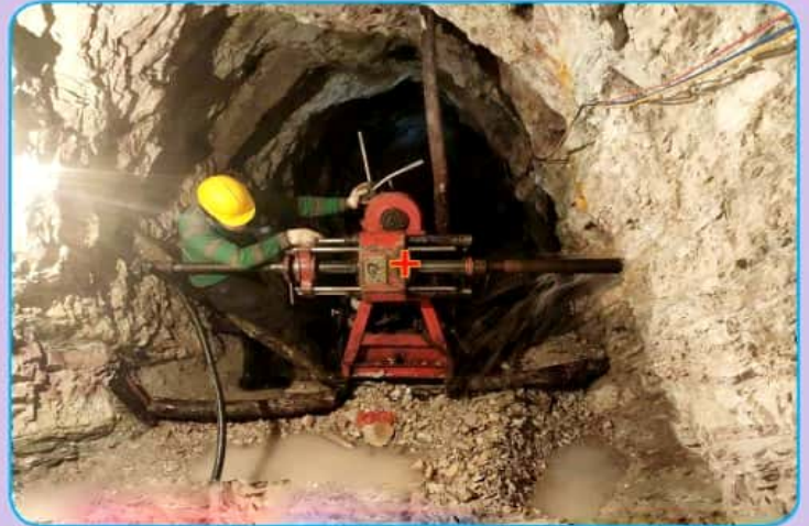
Horizontal Drilling inside Tunnel
