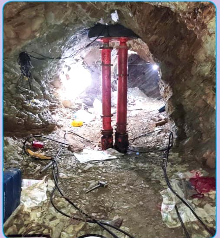
Plate Jacking Test inside Tunnel
