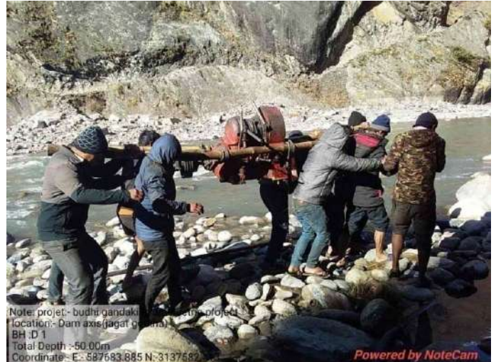
Fig: Manual carriage of the drilling equipment to the destination site
