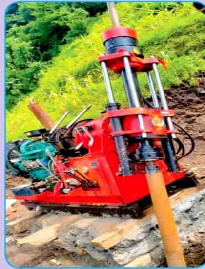
320m Rotary Drilling at KTFT Project with 1000m capacity Drilling Machine
