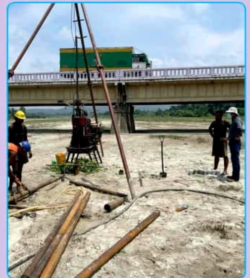
Field work Monitoring by Senior Geotechnical Engineer via Random Site Visit
